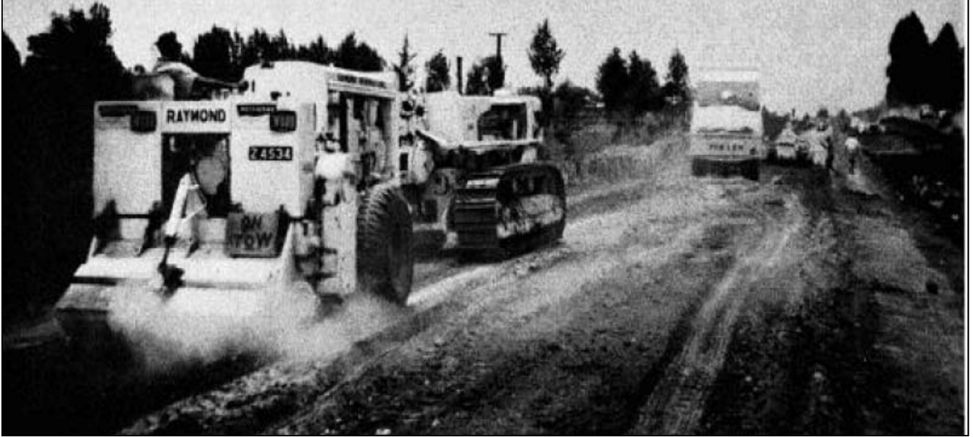
The Wood prepariser at work preparing for the sub-base of the road prior to stabilising
